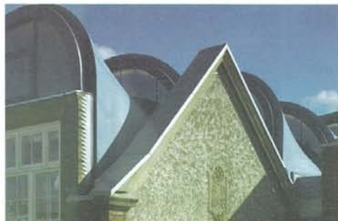
View of the clerestory lights which close the GRP ribbons.
